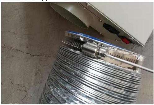
**STEP 2** Put the exhaust pipe on the product interface, tighten the fastening screws.
